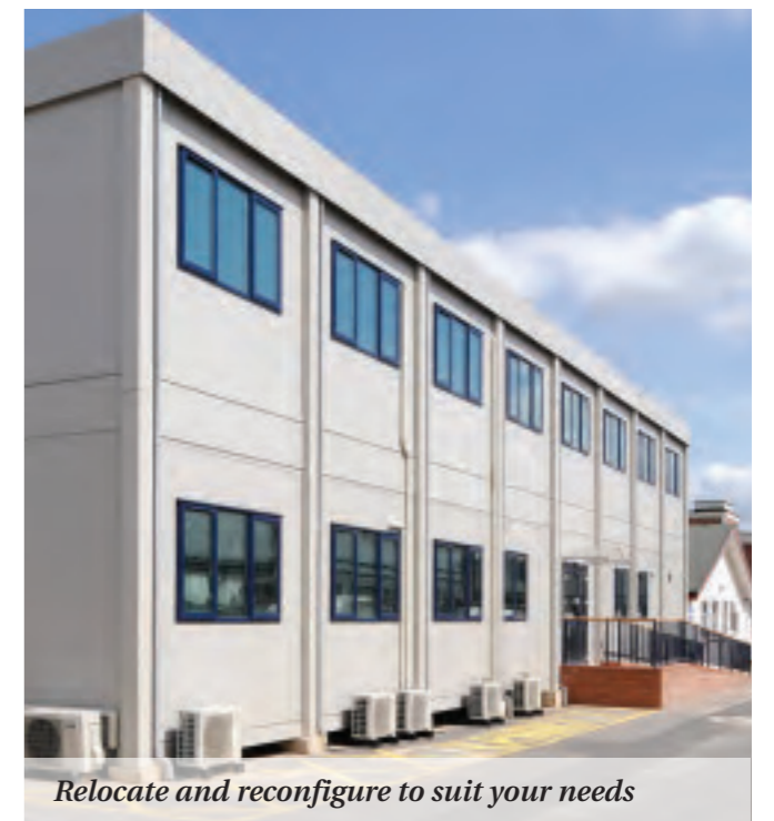
Office accommodation prior to relocation
