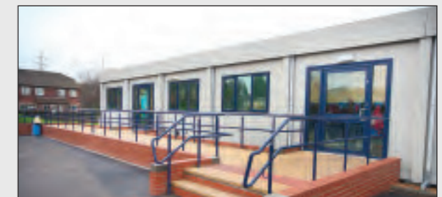
2012 – Classrooms in new locations converted from offices
